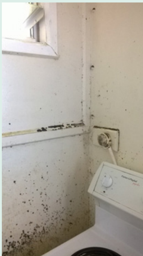
Figure 1. Mould in the kitchen of a house visited by a Well Homes housing assessor.
